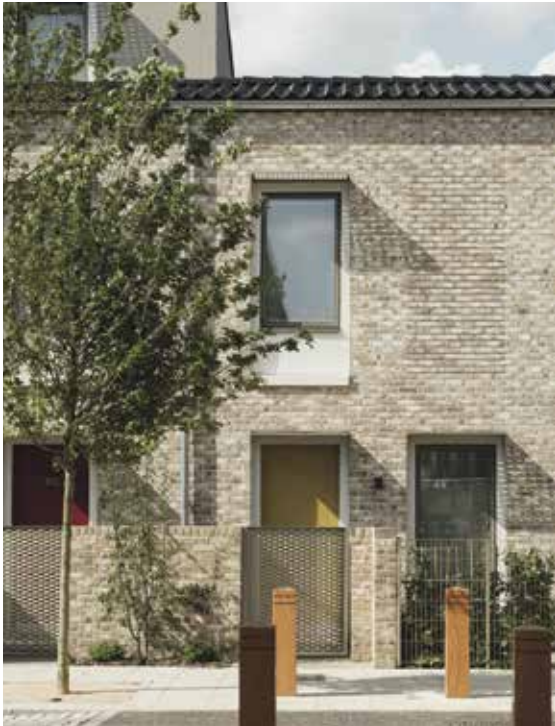
Crest's Belgravia Buff Multi and Grosvenor Multi, a mix of the two brick types created a bespoke and unique blend which complemented the Victorian terraced housing design.
