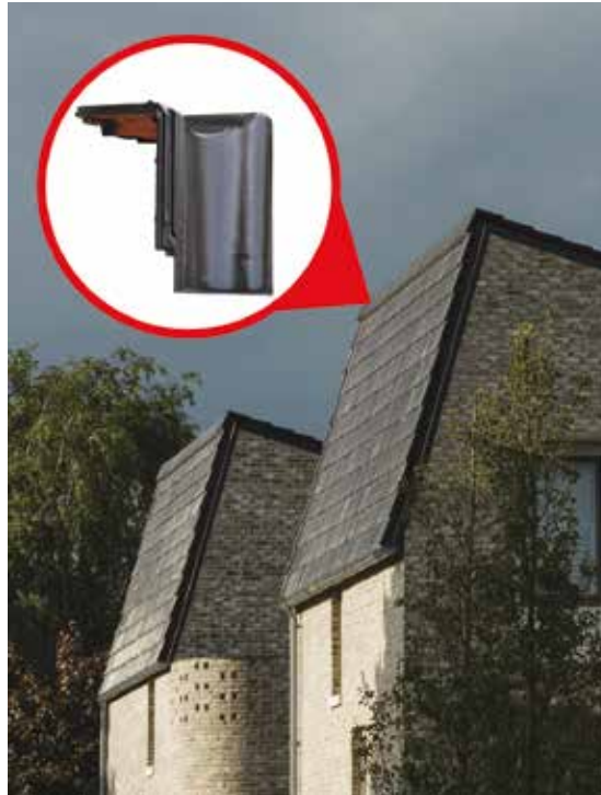
Crest Nelskamp specifically designed 70° angle H14 interlocking black gloss clay roofing tile. The unique roofing system flows without interruption continuously from eave to ridge.
